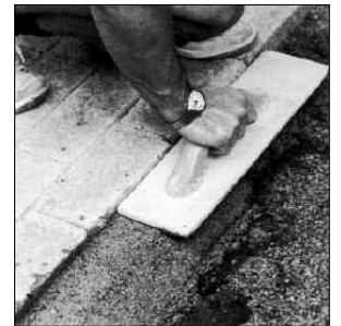
Concrete edge restraint using wooden float
