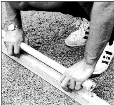
Using a screed board, spread the bedding sand to required levels.
